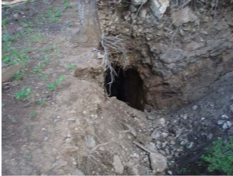
Photo#15 Dangerously open stope on the border of the Silver Dollar and 16 To 1 patented claims (B. Schuld 7/22/10).
