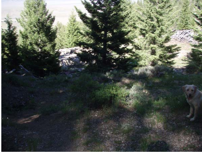
Photo #17 Looking down on waste dump and hoist house foundation of the Silver Dollar Shaft. (B. Schuld 7/22/10).
