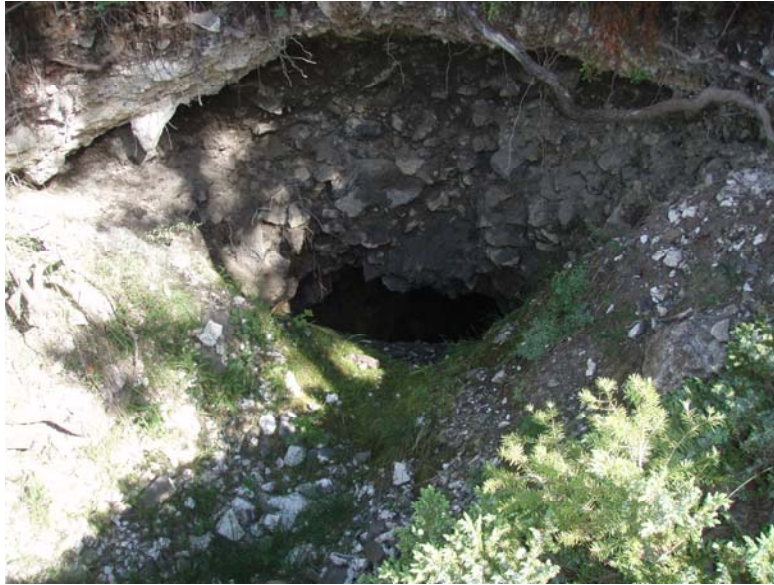
Photo#36 Dangerous opening of the Dorothy Tunnel adit. (B. Schuld 7/22/10).
