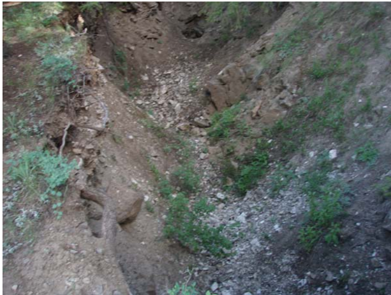
Photo #16 Caved Stopes and cross cuts extend from the open shaft on the west side of the Silver Dollar claim onto the 16 To 1 claim
