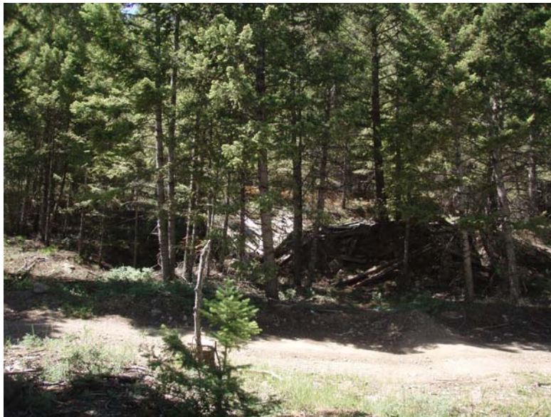
Photo #33 Caved adit for the Pittsburg-Idaho (P.I. Tunnel) (B. Schuld 7/22/10).
