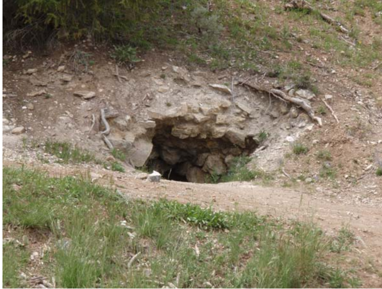
Photo #5 The Glen adit and tunnel are adjacent to the Meadow Lake public road. It was apparent that the public has and uses its access to enter and explore this dangerous mine opening. The Glen Waste Dump was sampled since public access traverse it, and although it was small, this sample may provide information about the typical constituents of mine waste in the Gilmore area. (T. Elayer 7/22/10)
