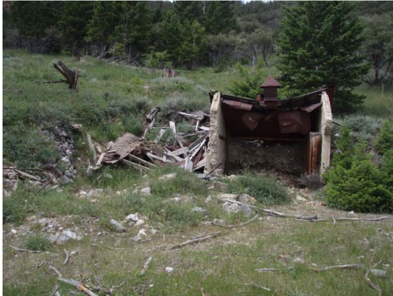
Photo #38 Concrete Dog House and Tunnel Adit on Andy Claim on north end of the "Old" Gilmore Town site.
