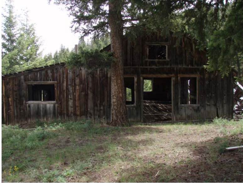
Photo # 46 Mining Office (?) in the "Old" Gilmore Town site. (B. Schuld 7/22/10).
