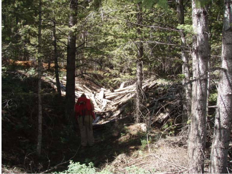
Photo #32 Caved adit for the Pittsburg-Idaho (P.I. Tunnel) (B. Schuld 7/22/10)
