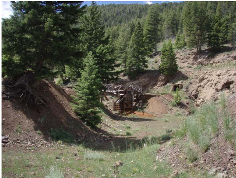
Photo #20 Three dangerously open adits remain on the Silver Dollar. There as apparently some redevelopment work that was conducted on these adits and a small ore bin/chute was constructed to ship some ore or samples (B. Schuld 7/22/10).
