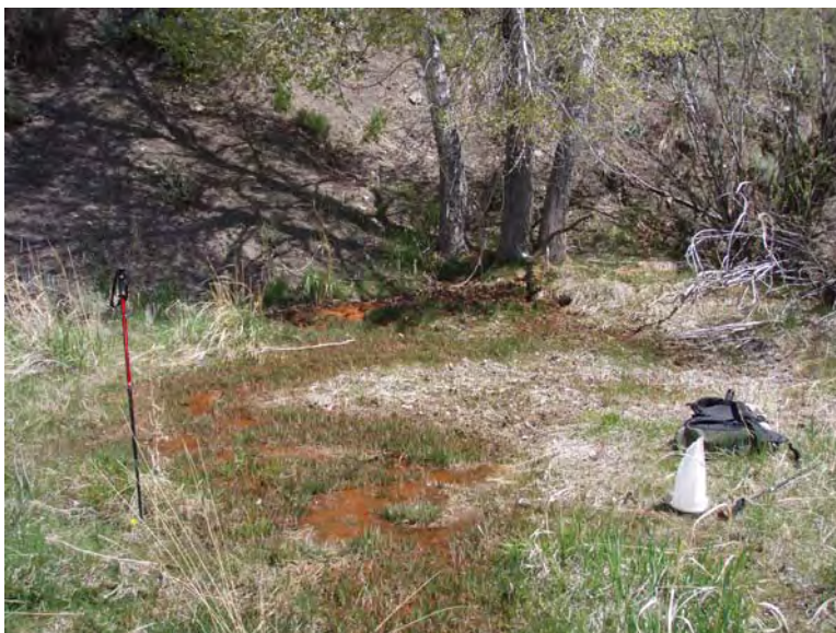
Minor drainage (approximately 1 gpm) flowing from the Bonanza Tunnel. Orange precipitates, prompted collections of IMWD6SW-1 (May 2007)
