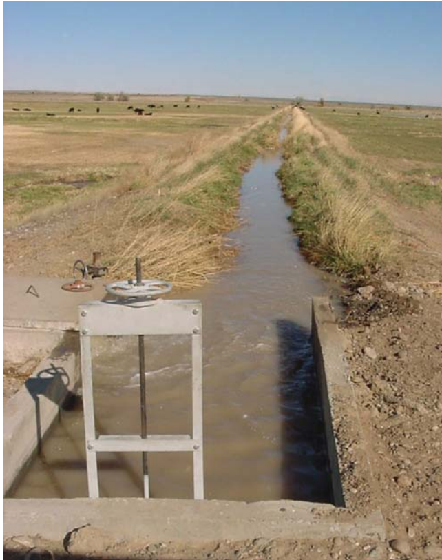
Figure 1. Potato processing wastewater being land applied to flood irrigation field.
