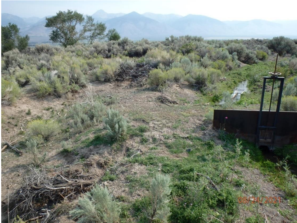
Figure D-3. Alternative view of the headgate along Lawson Creek. There is no flow path for water when the headgate is closed. The natural channel is to the left of the photo. There is ample evidence of soil disturbance suggesting heavy machinery is often used to manipulate the stream channel.
