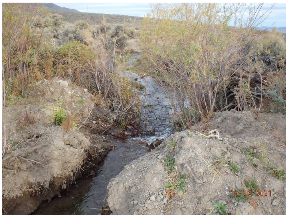
Figure D-6. Headcut caused by moving Lawson Creek in and out of the natural channel to deliver water to the headgate and downstream overwidening.
