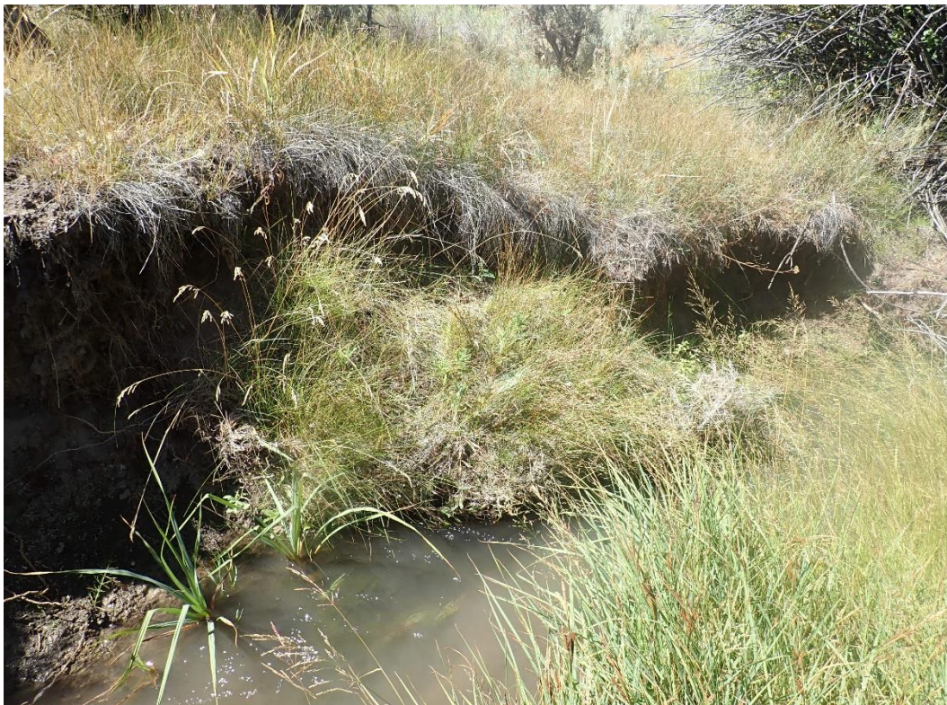
Figure D-15. Bank collapse and high-turbidity water along Burnt Creek.
