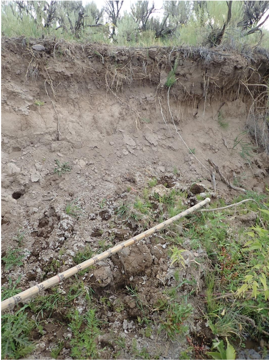
Figure D-8. Bank trampling and large cutbank along Lawson Creek.
