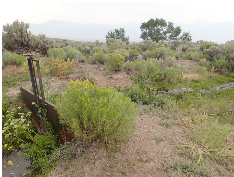
Figure D-2. Flow from Lawson Creek diverted through a headgate per Idaho water right 73-79.
