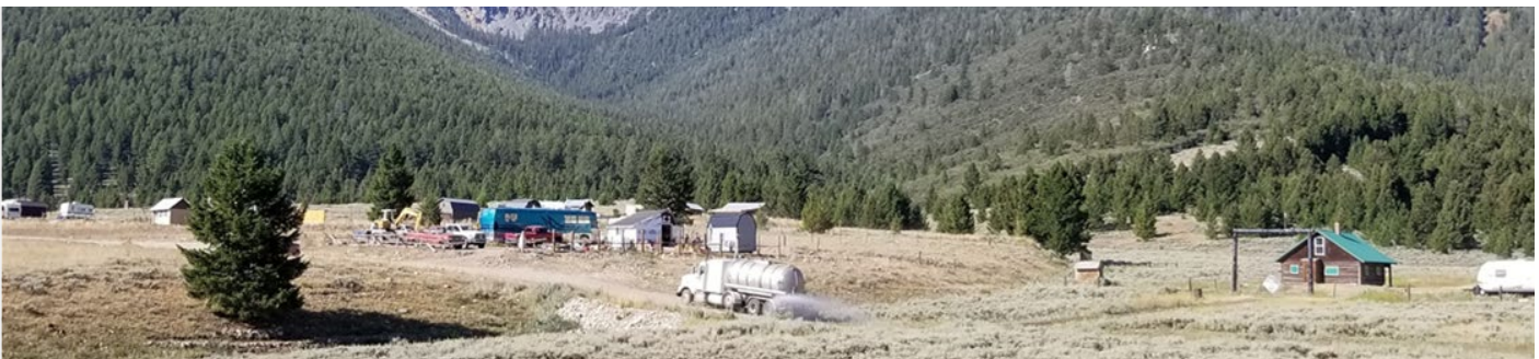
A tanker truck traveling south on Quartzite Avenue at the Gilmore townsite sprays water on the rights-of-way prior to applying magnesium chloride. Photo credit: Kevin Kostka, August 17, 2023
