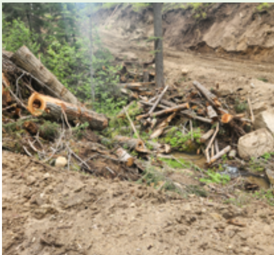
Figure C16. Dirt sidecast into the SPZ.
