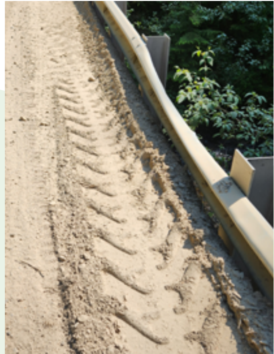
Figure C15. Dirt graded off edge of bridge.
