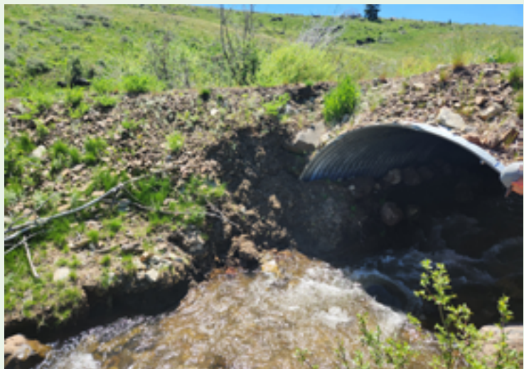
Figure C6. Erosion of the fill.
