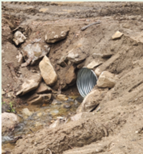
Figure C5. Short culvert pipe, vertical headwalls.
