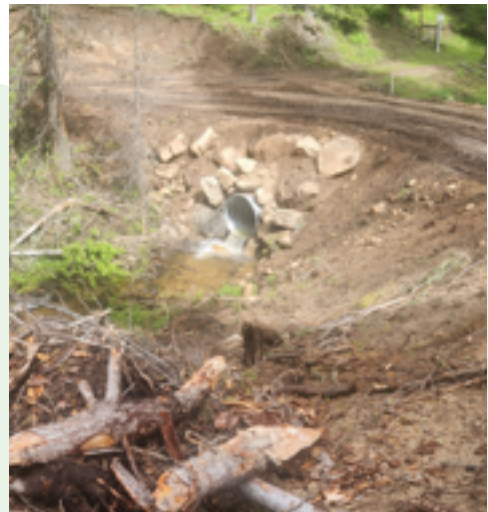
Figure C4. Perched culvert pipe and bare unstable dirt.
