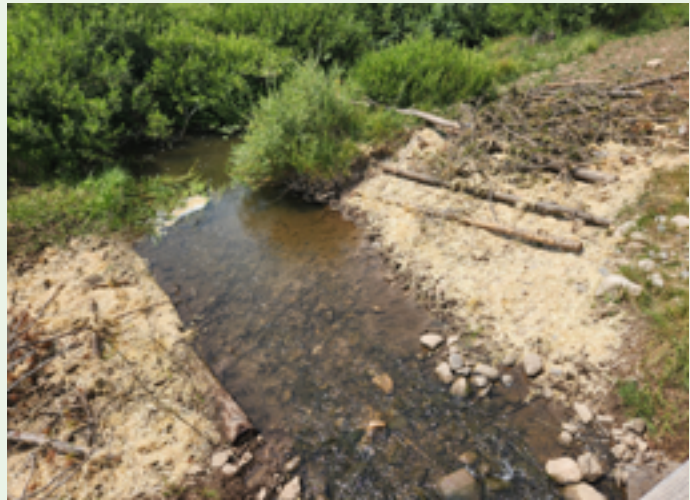
Figure C11. Stream crossing protected by slash.
