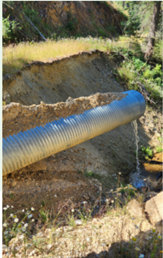
Figure C8. Blown out culvert (blocked by slash).
