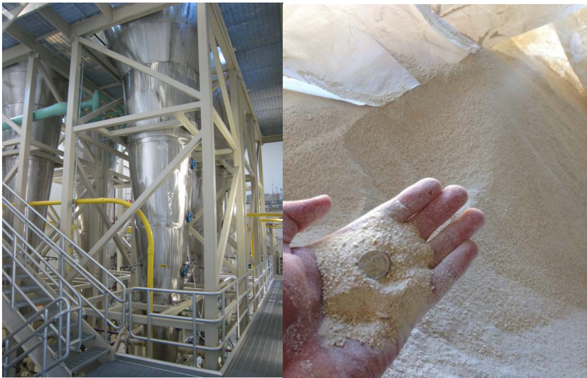
FIGURE 1. CITY OF BOISE STRUVITE PRODUCTION FACILITY REACTORS (LEFT) AND STRUVITE (RIGHT).
