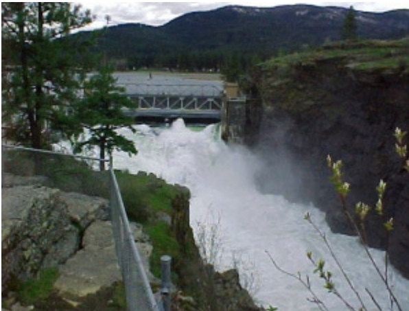
Avista Dam: Photo courtesy City of Post Falls
