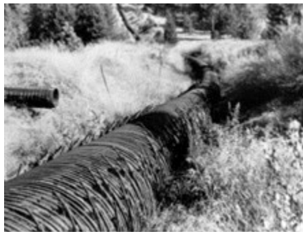
Wooden pipe: North Idaho Museum photo
