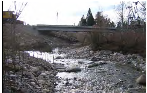
The Targhee Creek crossing at Highway 20 after construction. The impassable culvert was replaced by a fish-friendly bridge.
