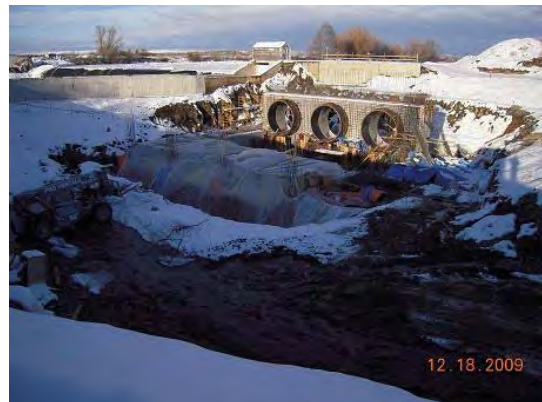
Construction of Dam
