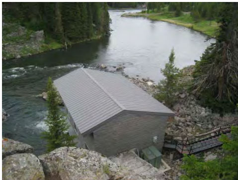
Buffalo River Powerhouse
