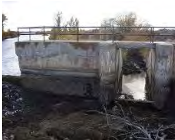
View of Old Dam
