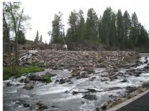
Newly constructed Fish Ladder
