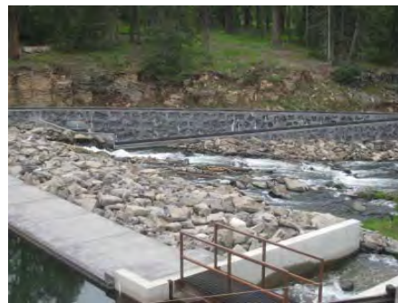
View of Raceway
