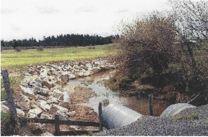
Figure 7. Streambank stabilization (rock riprap).
