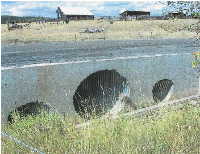
Figure 6. Newly installed culvert.
