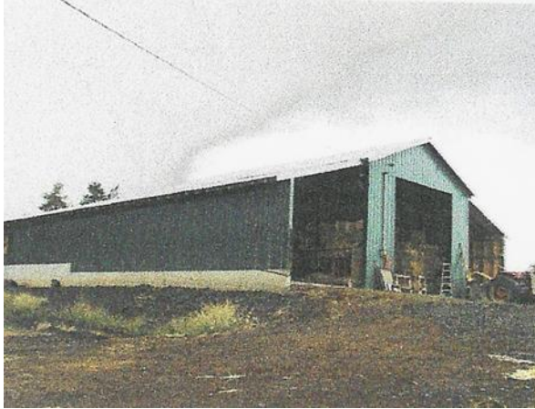
Figure 10. Barn complex after feedlot restoration project.
